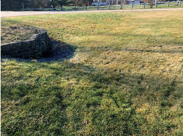
29 Gundalow - 1 (Drainage Area)
